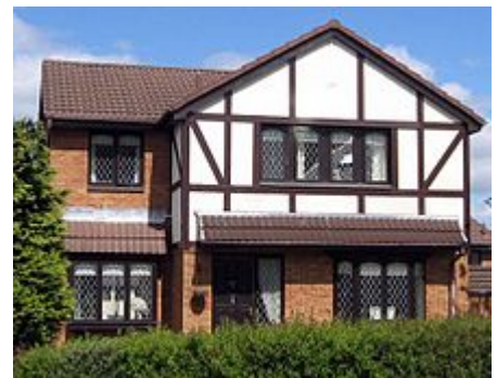
"A modern Tudorbethan" house with uPVC gutters and downspouts, fascia, decorative imitation "half-timbering", windows, and doors
